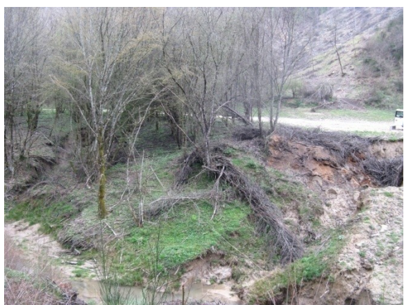
Alluvial terrace reworked by gully erosion (Pietrasecca)
