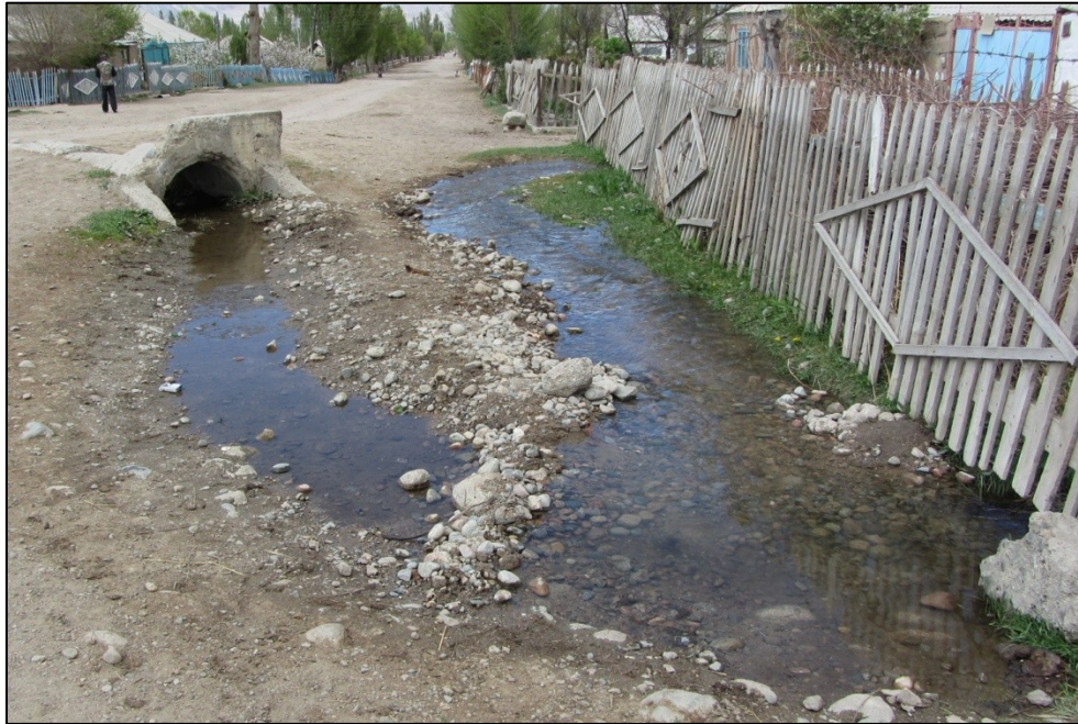
Figure 33: Irrigation channel with a diverting trench into a garden (Photo: Topbaev, May 2012).
