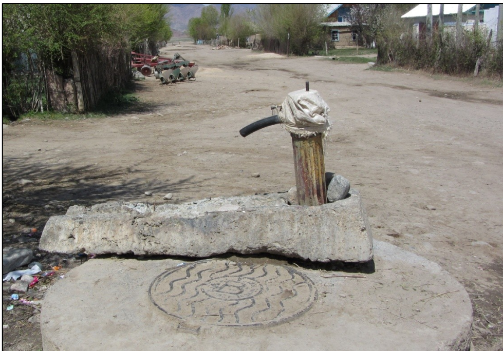
Figure 17: Standpipe in the street of Kara-Suu (Photo: Topbaev, April 2011).
