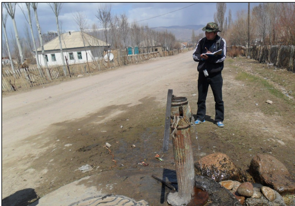
Figure 15: Visual defining of the pump's condition in Kara-Suu (Photo: Kasymov, April 2011).
