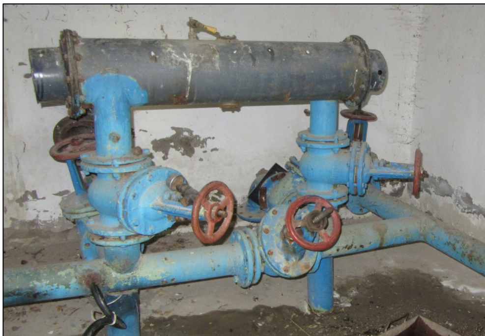
Figure 23: The non-working quartz filter in the groundwater pump station of Kara-Suu (Photo: Topbaev, August 2012).
