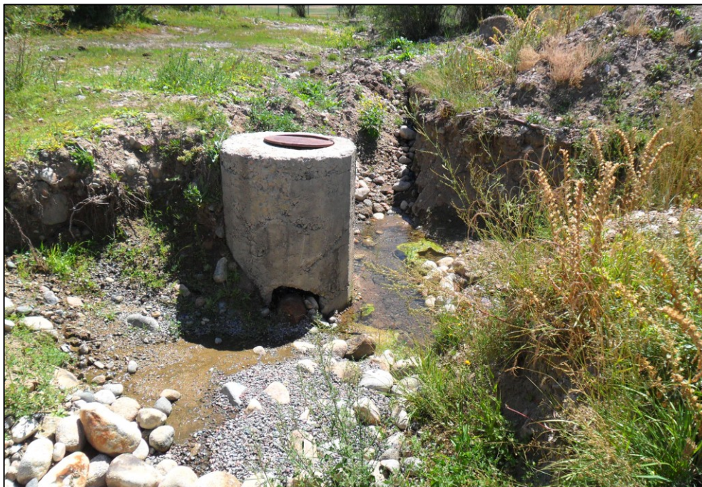
Figure 29: Well of the Swamp Drainage System after a reconstruction process (Photo: Kasymov, August 2011).
