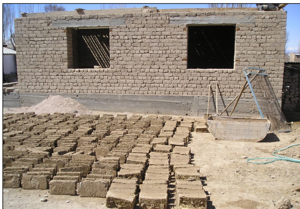
Figure 37: Drying of adobe bricks for construction work (Photo: Topbaev, April 2011).
