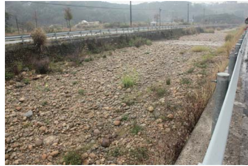
Figure A5. A modernized channel in the box-shaped valley in the Tungxiao River catchment (location: 24°27'20.90" N, 120°44'6.72" E; facing west, 25 December 2014). The tableland segments in the background of this photo are classified as the ST. The valley floor is classified as AL; the fluvial channel is constrained by the artificial levees and covered by abundant gravel and cobble depositions.
