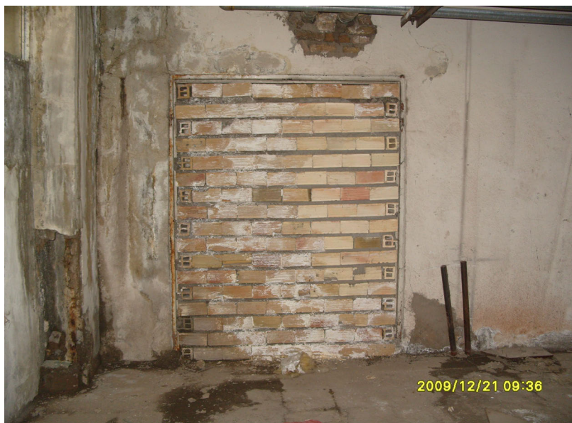
Fig. 4 Building X, basement, the bricked doors of basement rooms.
