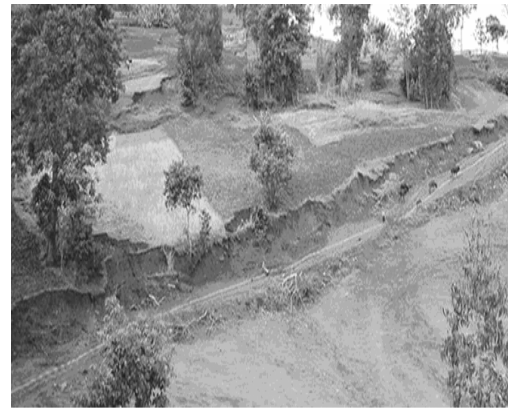
Figure 24: Soil erosion damage – Talus edge along the road.
