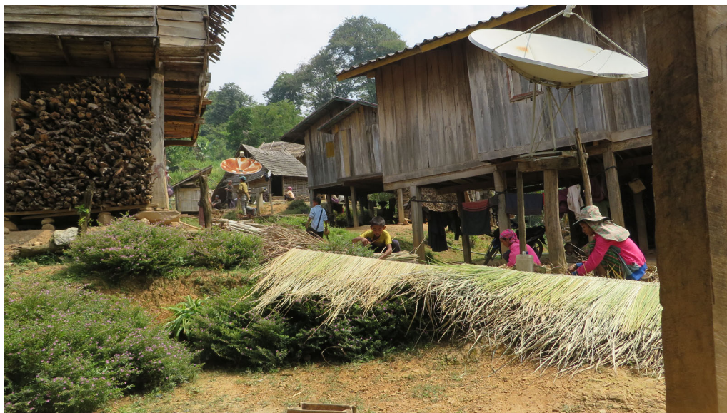
FIGURE 4 The women of the neighborhood make the thatch for the roofing of a newly erected bamboo house. (Photo: Author, 2014) A view up a village path flanked by timber houses. Women are sitting on the path, tying cogongrass to bamboo sticks to prepare thatch. [This figure appears in color in the online issue]
