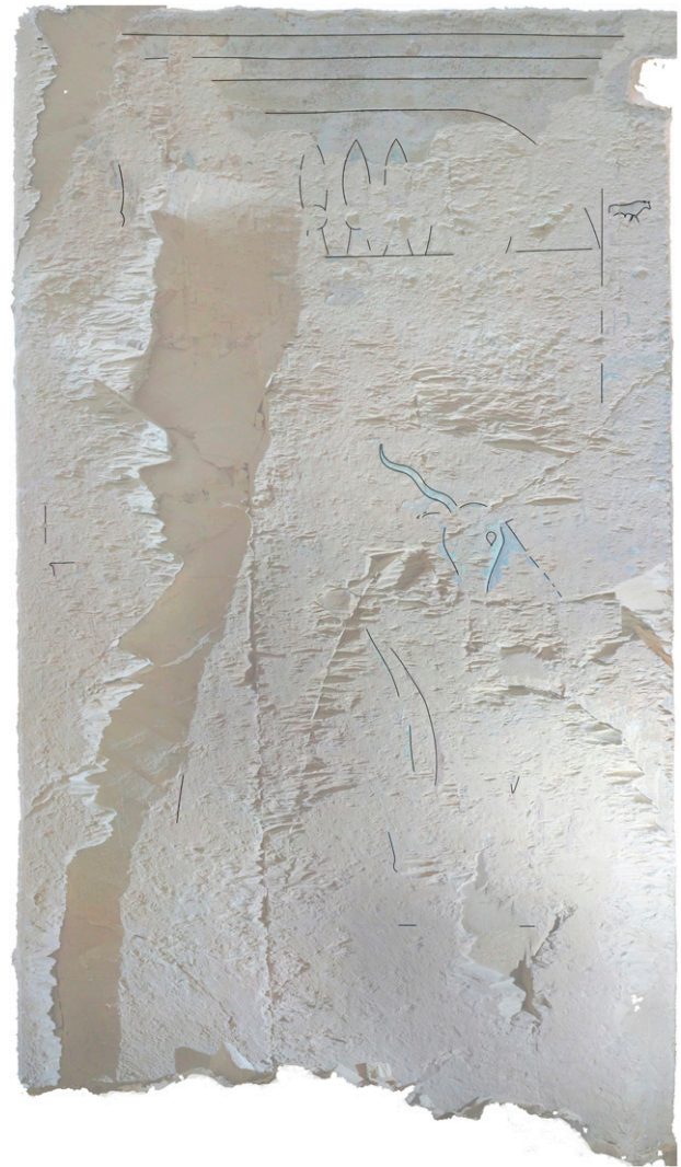
Fig. 6. Orthophoto of the east half of the south wall of room I. Provisional tracing of the remains of the decoration (orthophoto and drawing: W. Hovestreydt).
