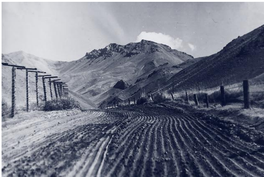
Figure 4.5 The Control-Track Strip in combination with fence on the right to prevent ‘false signal’ due to wild species. The border zone in Erkechtam area in 1979
