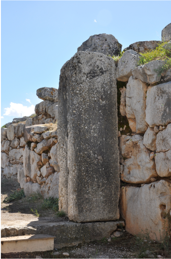
Fig. 10 Tiryns conglomerate block of the Main Entrance (9.6 tonnes). Discussed and calculated together with other conglomerate blocks from Tiryns in Brysbaert 2015a.
