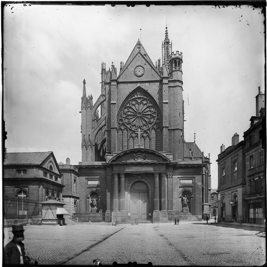
Fig. 5 | Metz, Southern facade of the cathedral, Changes made in neo-Gothic style, late 19th century.
