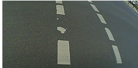
(f) Missing line segment.
