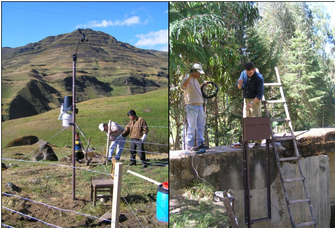
Figure 1–1: During the CASCUS research project, three Davis Vantage Pro II weather stations and two pressure transducers (OTT Orpheus Mini) were installed in the area under investigation. Left: Installation of the Alto Chetilla rain gauge at 3422 m asl. Right: Installation of the pressure transducer at the Ronquillo water intake at an altitude of 2838 m asl. To view sites composing the hydro-meteorological monitoring network, refer to the maps in Figure 2–1 and Figure 5–1 (Photos: Krois 2009).
