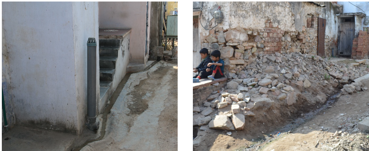
Fig. 44: Left: Ventilation pipe of latrine and open pucca drain for grey water. Right: Grey water flowing on the street without a pucca drain, Khara Kuaa 2017.
