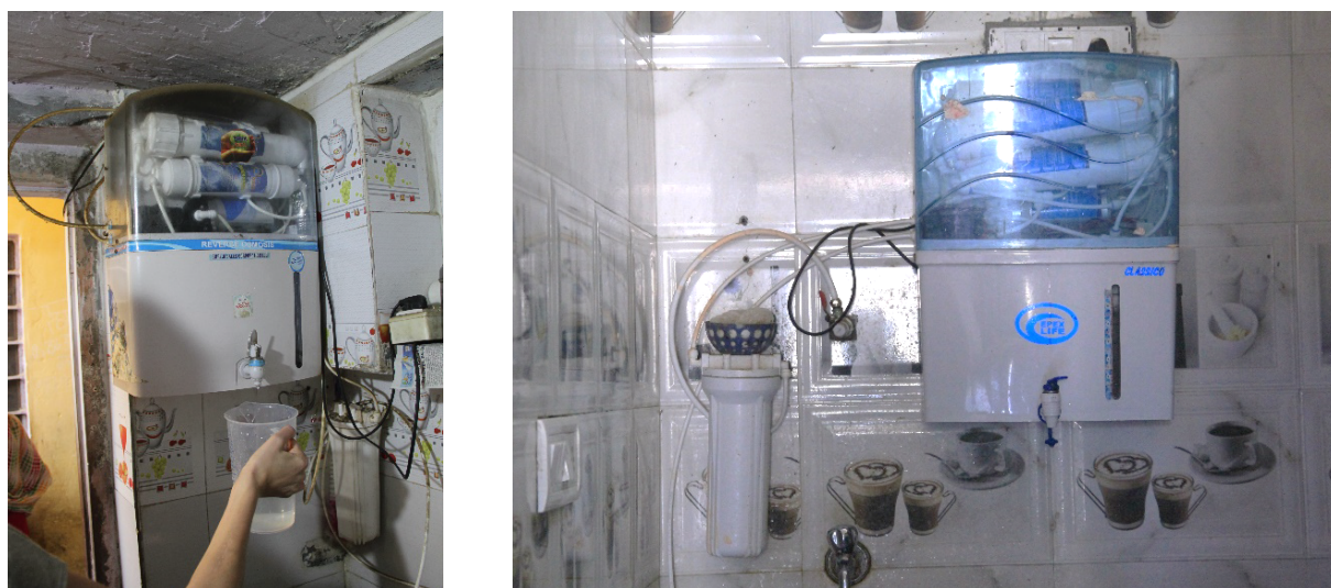
Fig. 36: Sampling of domestic RO systems in Nai Ki Thari, November 2016. Left side: Sample taken at the RO tap. Right side: Typical RO system with a pre-filter unit (left) and the main RO unit (right).
