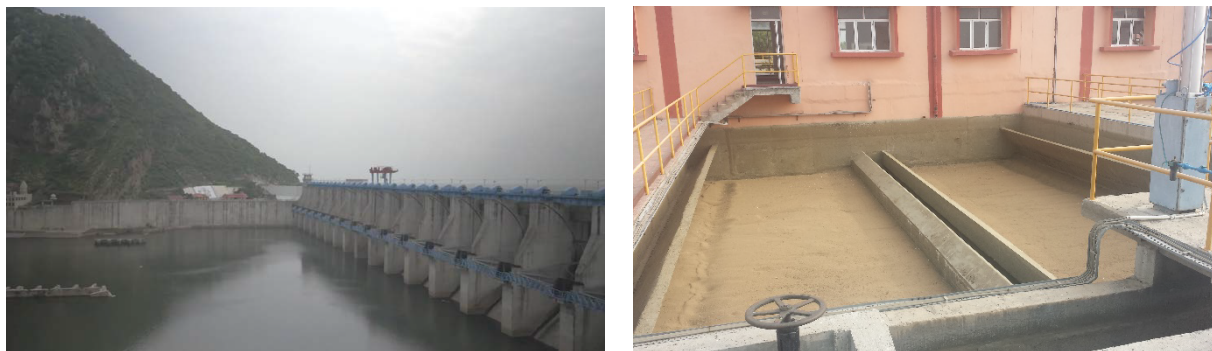
Fig. 35: Bisalpur reservoir 110 km south of Jaipur. water supply system. Left: Dam. Right: Sand filtration unit at Surajpura Water Treatment Plant., 2017.
