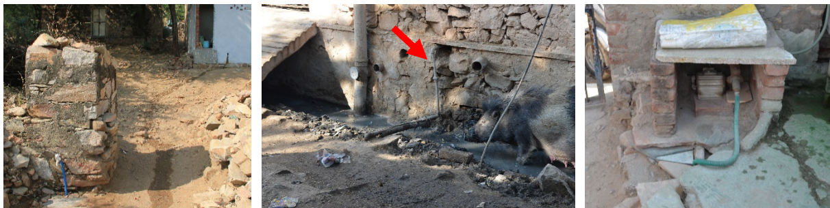
Fig. 37: Diversity of water line connections within Khara Kuaa. Left: Tap shared by several HHs. Middle: Pipe going, above the open drain, into a house. Right: Some HHs attached (illegally) a pump to their water connection to get more water out of it. Here, it is a small stone factory.
