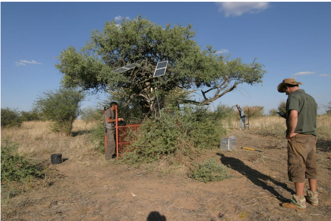
Figure 4: The author sending test commands via GSM-network to the trap. Solar panels supply power and charge the 12V battery.
