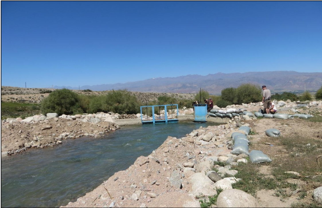
Figure 32: The Ukok-Kairma weir in 2013. On the right of the weir are sand bags, which protected the system from a flood event a few days ago (Photo: Kasymov, 2013).
