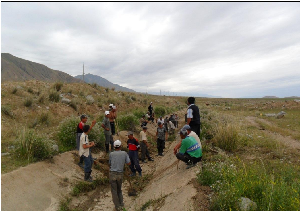
Figure 29: Farmers removing sediment from the Topon-Aryk canal section near the mountains (Photo: Kasymov, 2010).
