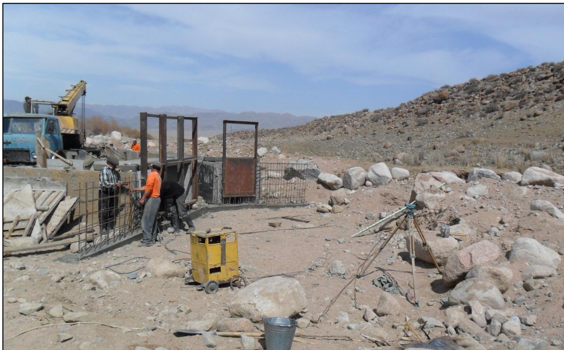
Figure 31: Rekonstruktion of the Ukok-Kairma weir after its destruction by a debris flow in August 2010 (Photo: Kasymov, 2010).
