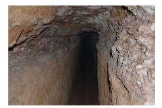
Fig. 12 The *adit* at Bureta is some 100 m long, 2 m high and 0.9 m wide.
