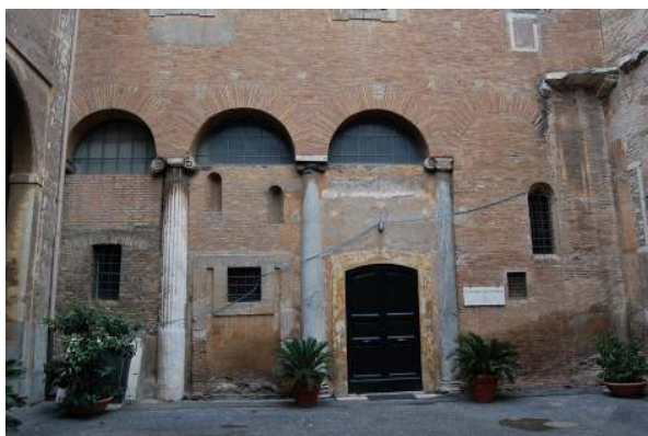
Fig. 20 SS. Quattro Coronati: remains of the first phase nave colonnade set into the later phase courtyard.
