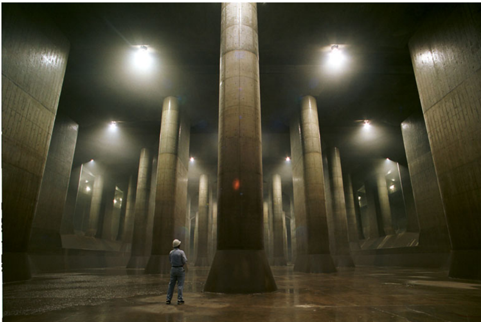
Figure 2. Critical infrastructure: G-Cans, Tokyo is an underground infrastructure for prevention of flooding during rainy season (Source: G-Cans project, Tokyo [ http://www.g-cans.jp/ ]).
