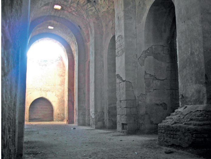
Fig. 25 | Large cistern, view to the east.
