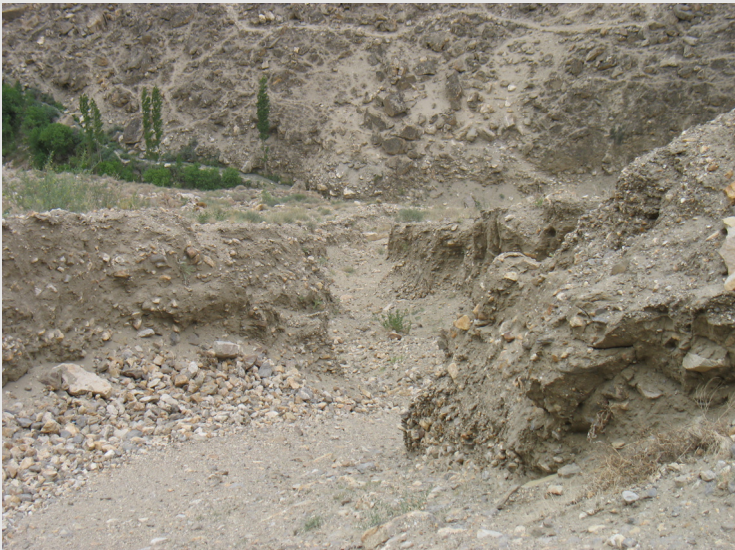
Environmental damages below the power channel Photo: Author, May 2008
