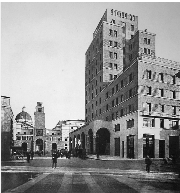
Figure 26: M. Piacentini: Rear side of the INA tower, Brescia, 1932 (FPF, ff. 64.2).
