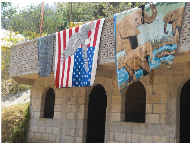
Figure 5.3: Site construction of Marco's new house
