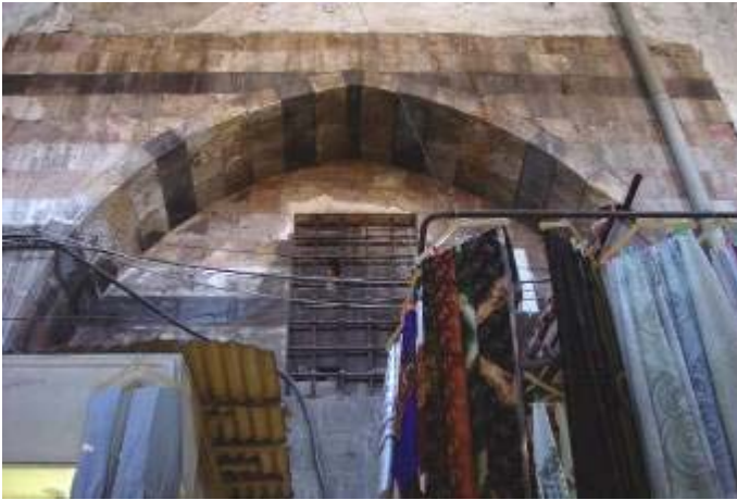
Abb. 596: Portal Ḥān al-Marādniya (Weber)
