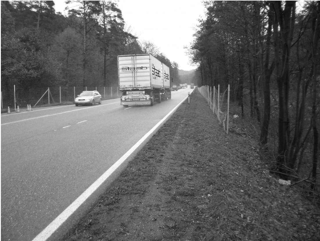
Figure 7. The partly fenced B10 with 3 lanes and high traffic volume of up to 25 000 vehicles/day cuts the forested mountain range of Northern Vosges and Palatine Forest in two.
