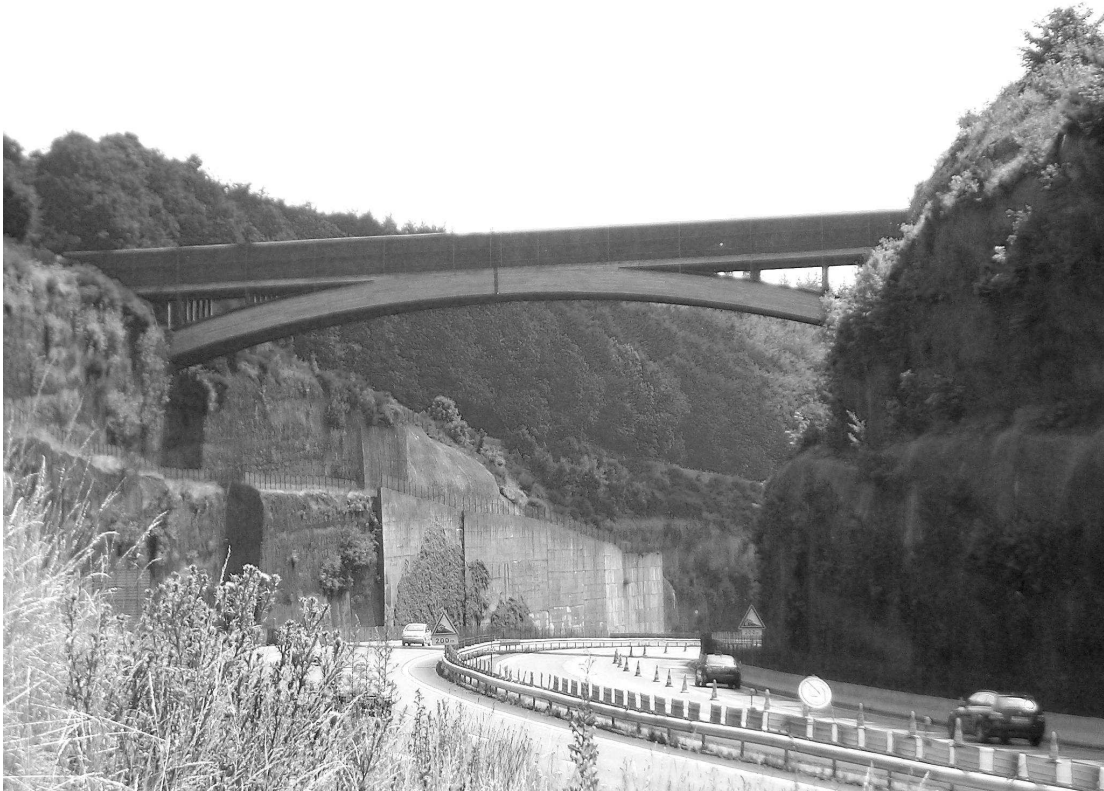
Figure 3. A major barrier to wildlife: The French motorway A4 at “Col du Saverne / Zaberner Steige” where the mountain range of the Northern Vosges narrows and connects to the Central Vosges. The wildlife overpass of 9 m width and 57 m length was closed for wildlife several years ago to stop the spread of swine fever.
