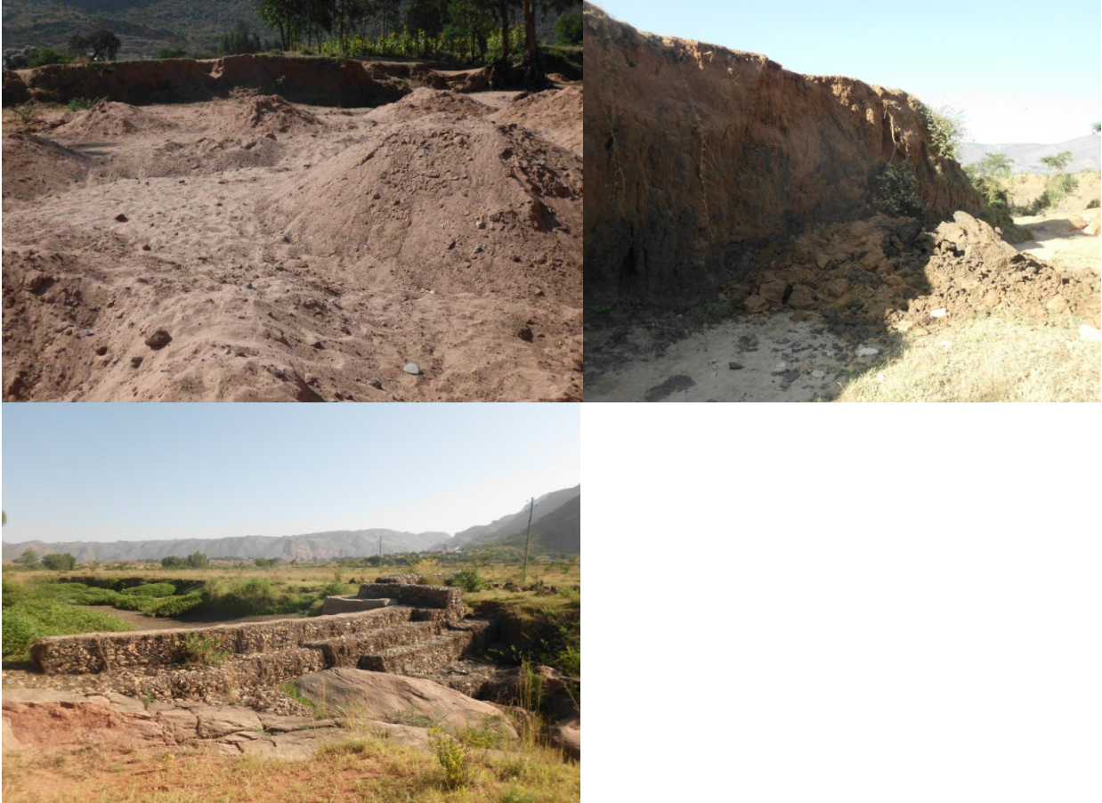
Figure 4-36: Above left: Sand quarry on stream bed, Above right: Stream bank instability and Below left: Gabion work across stream.
