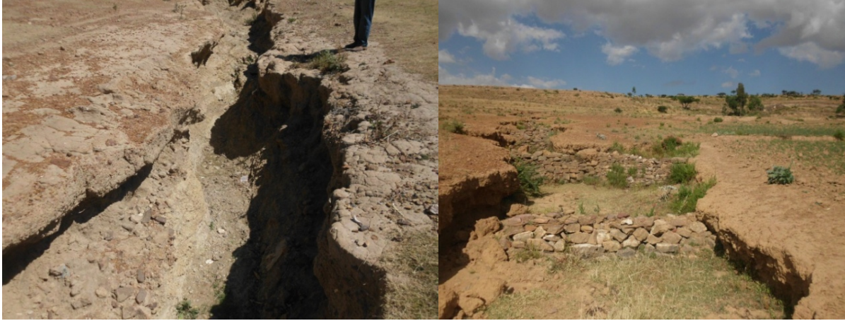
Figure 4-30: Gully formation on the colluvial zone in the Tsenkanet study site.
