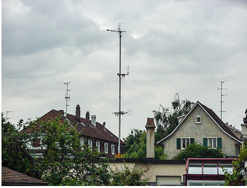
a) Tower in a vegetated backyard in Allschwil (ALLS)
