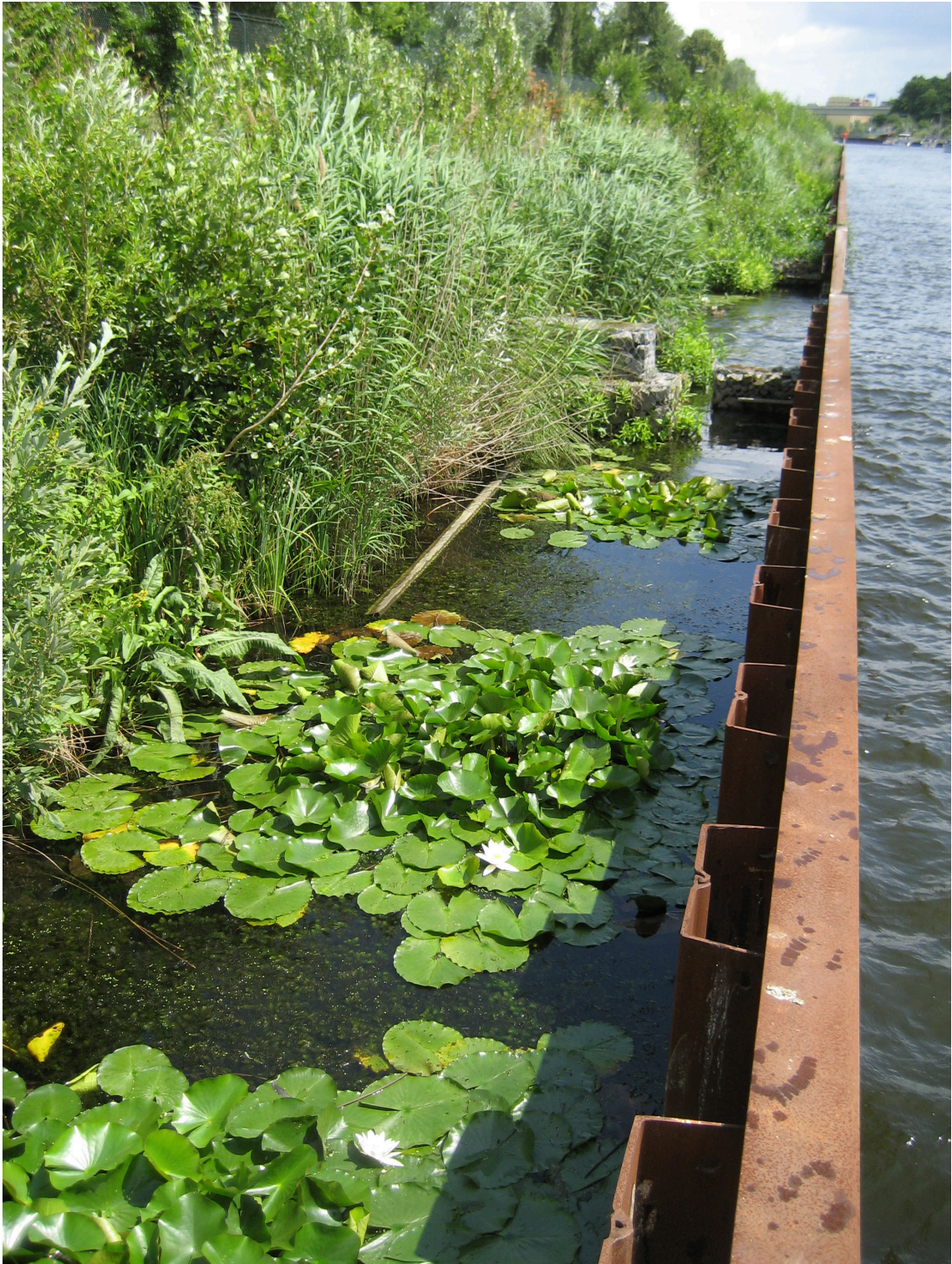
Figure 3.5: Dense vegetation inside the rehabilitation structure at the River Spree on the 6 th of July 2009.
