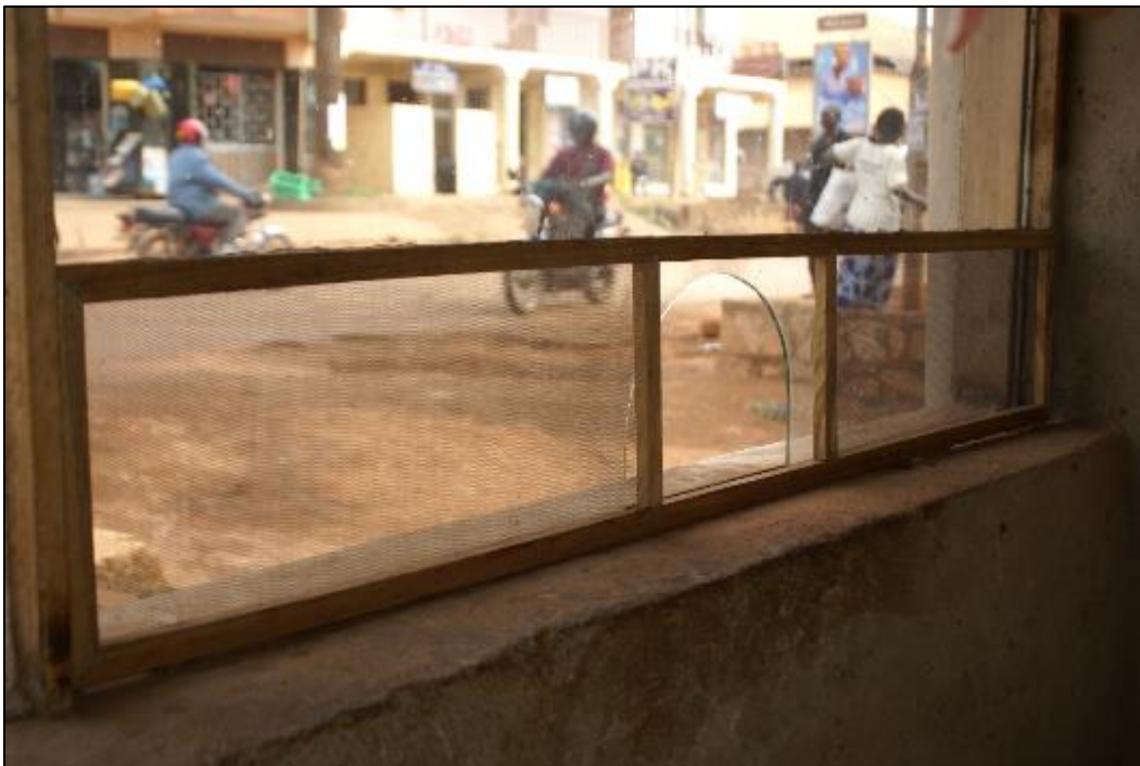
Figure 10 Pork joint from intervention with a net frame at the bottom of a glazed butchery © Martin Heilmann, ILRI / Freie Universität Berlin
