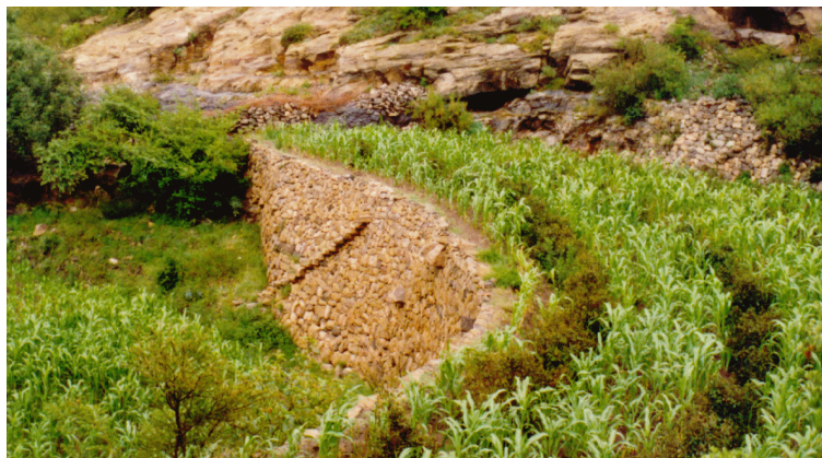
Photograph 4.4 House wall type of terrace (August 1997). The terrace wall is vertical and includes stairs to connect the upper and lower terrace. On both fields sorghum was grown, on the upper one with qat intercropping.
