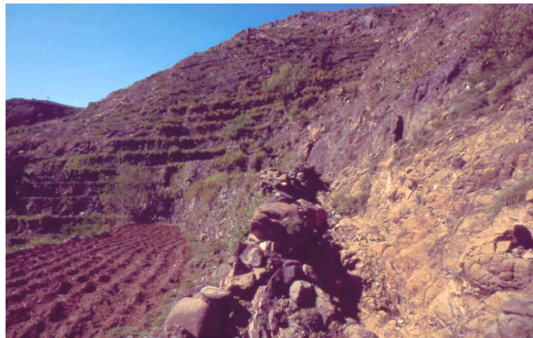
Photograph 4.1 Semi-pervious channels (in the center of the photo) protect the terraces (on the left) from destructive floods which come from the water harvesting areas (on the right). On the terraces, the plowing creates a corrugated pattern to increase retention.
