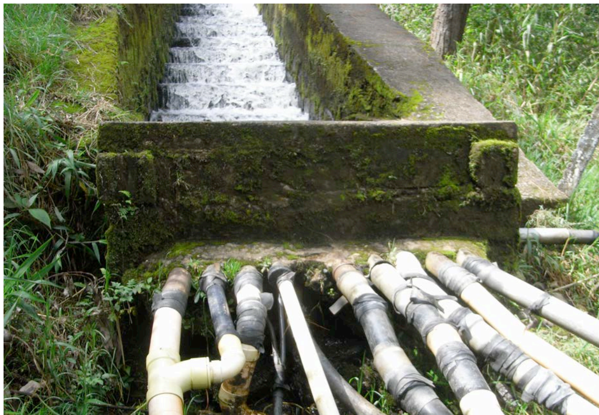
Figure 30 Alternative infrastructure built by inhabitants of Bello Oriente to capture raw water that overflows a tank of the company
