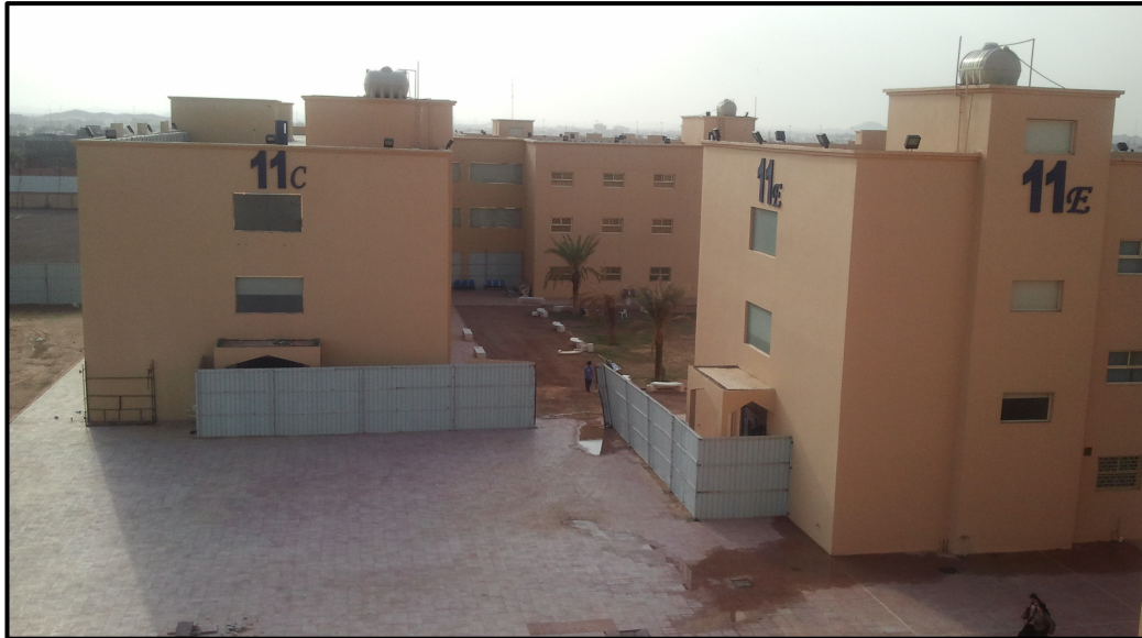
Figure 13. – The new Hail campus, during the finishing stages of construction
