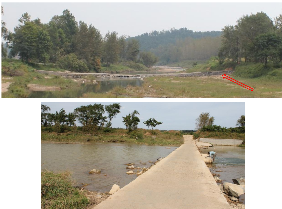
Figure 3.7 Small dam across the main channel in the Baocun watershed. The small dam affects the daily river discharge slightly, but the sediment load significantly, which intercepts sediments.
