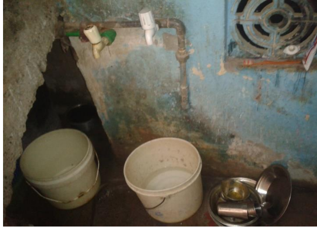
Figure 11: Two Taps are common in many Households; one is from municipality (could be illegal) and another is from bore well.
