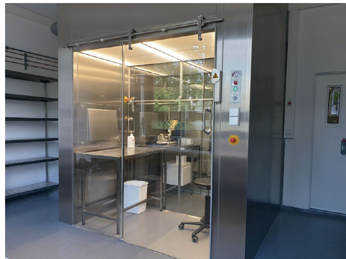
Fig. 3 | The Laminar Air Flow (LAF) cabinet. The LAF cabinet serves as a sterile intervention room for procedures involving Wildling mice and as an air lock to export samples from the Wildling area. Credit: Anke Lohan
