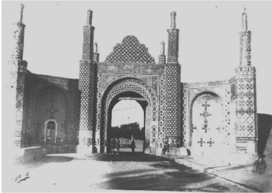
East . West view of Shemiran Gate in North of Tehran
