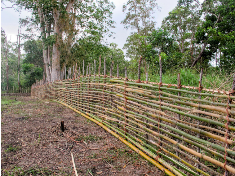
Figure 2.9: A newly constructed garden fence ( ηarake )
