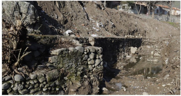
(b) River bank stabilization walls
