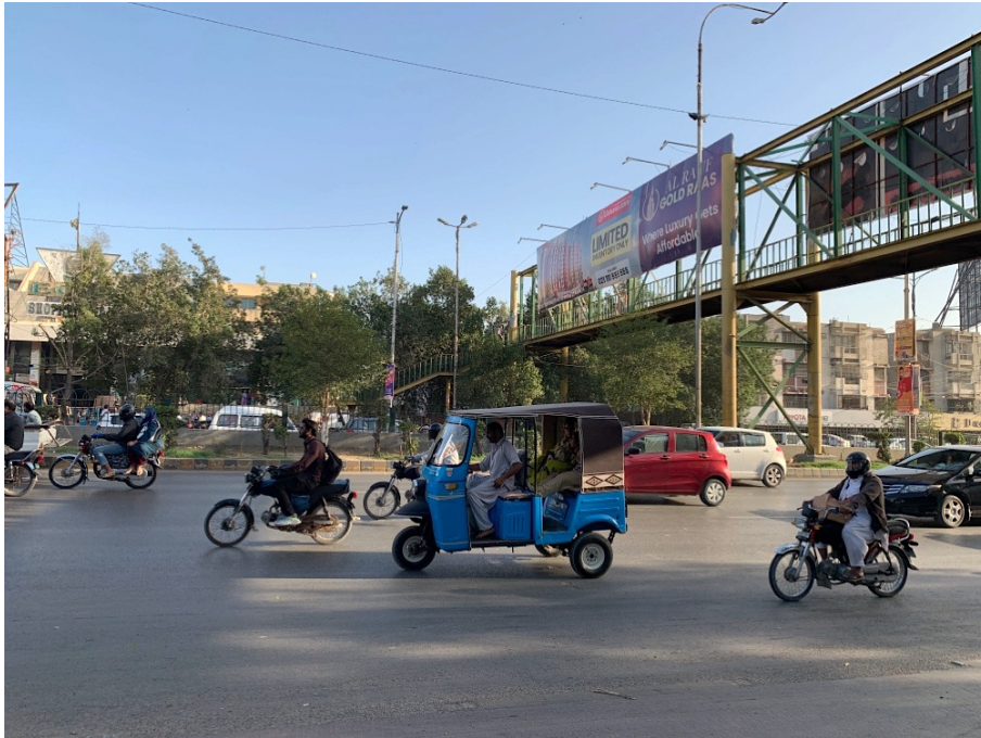
Figure 3. Pedestrian bridge at Shah-rae-Faisal Road.
