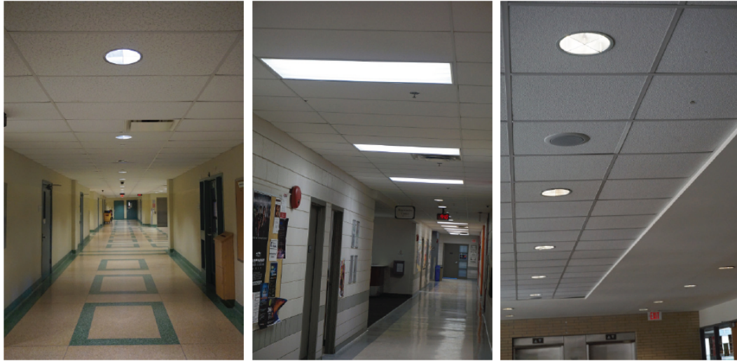
Figure 8.1: The arrangements of the ceiling lamps can be used for walking speed estimation
