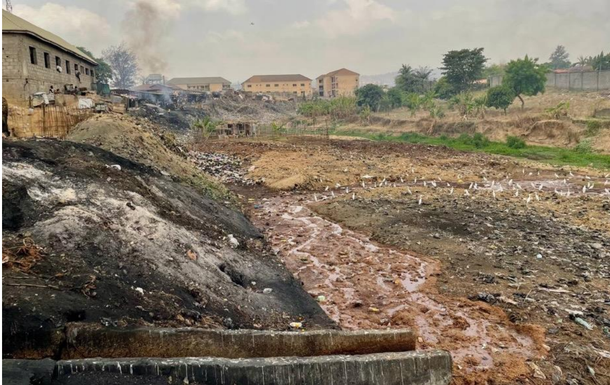
Figure 203: Main drainage spilling its contents into the streambed, digging a path into the ground until it reaches the stream.
