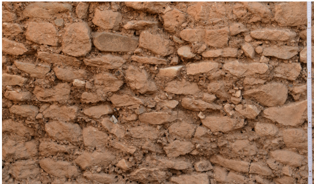
Figure 15: Reused materials in the mortar: bone, lithics, small stones, charcoal, and lime. Northern wall Loc. L9-80-23 of Room 16, area L9-80 (detail) (photo: Moritz Kinzel/DAI).
