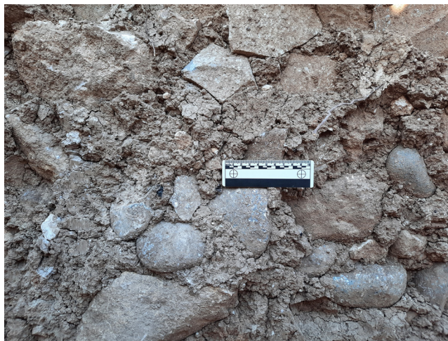
Figure 12: Boncuklu Tarla: Building GD4, close up of mud mortar with embedded river pebbles. (Photo: M. Kinzel, 2021, DAI-IST).
