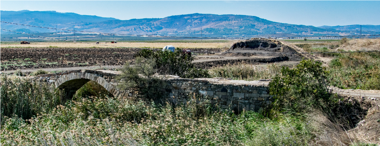
Fig. 5.1.4 Hacismail Köprüsü (bridge 4) in the western lower Bakırçay Valley.
