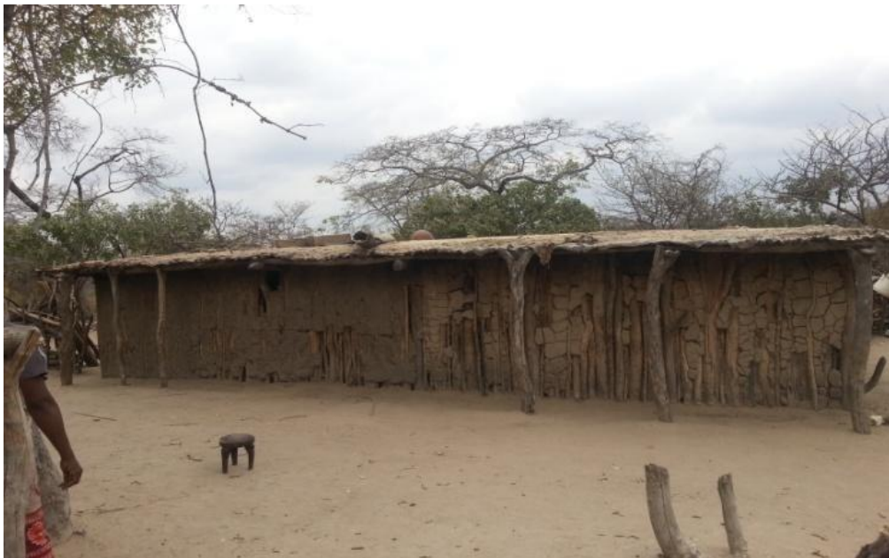
Figure 2.2: Tembe , a traditional Sandawe house (Photo by Anitha Tingira, 2015)
