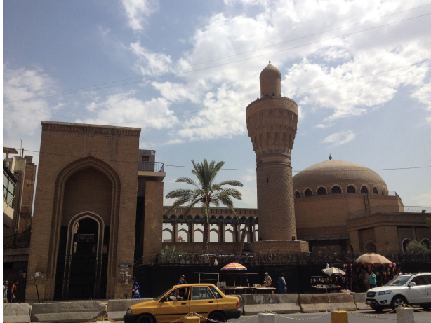
Fig. 1.4: Masjid al-Khulafā' (The Caliphs' Mosque) with the Ilkhanid Minaret, 2014
