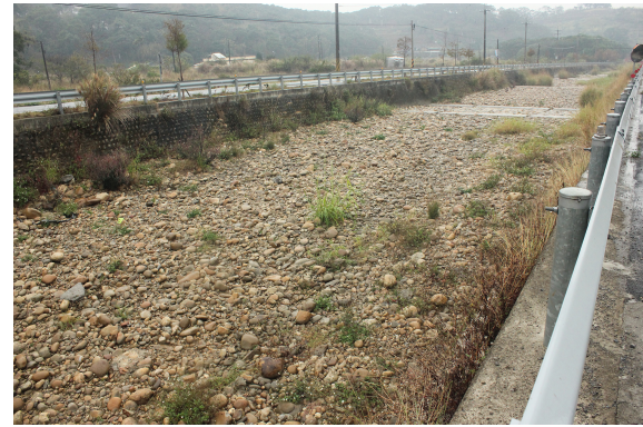
Figure A5. A modernized channel in the box-shaped valley in the Tungxiao River catchment (location: 24^{\circ}27'20.90'' N, 120^{\circ}44'6.72'' E; facing west, 25 December 2014). The tableland segments in the background of this photo are classified as the ST. The valley floor is classified as AL; the fluvial channel is constrained by the artificial levees and covered by abundant gravel and cobble depositions.
