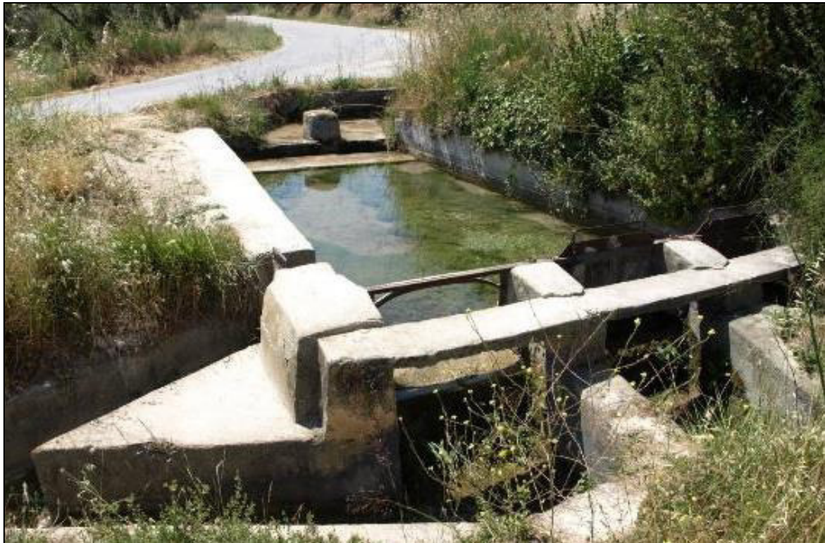
Fig. 3: Sluice gates and sedimentation basin in front of the inlet of the Balsa Alara reservoir (for the location, see Fig. 10).
