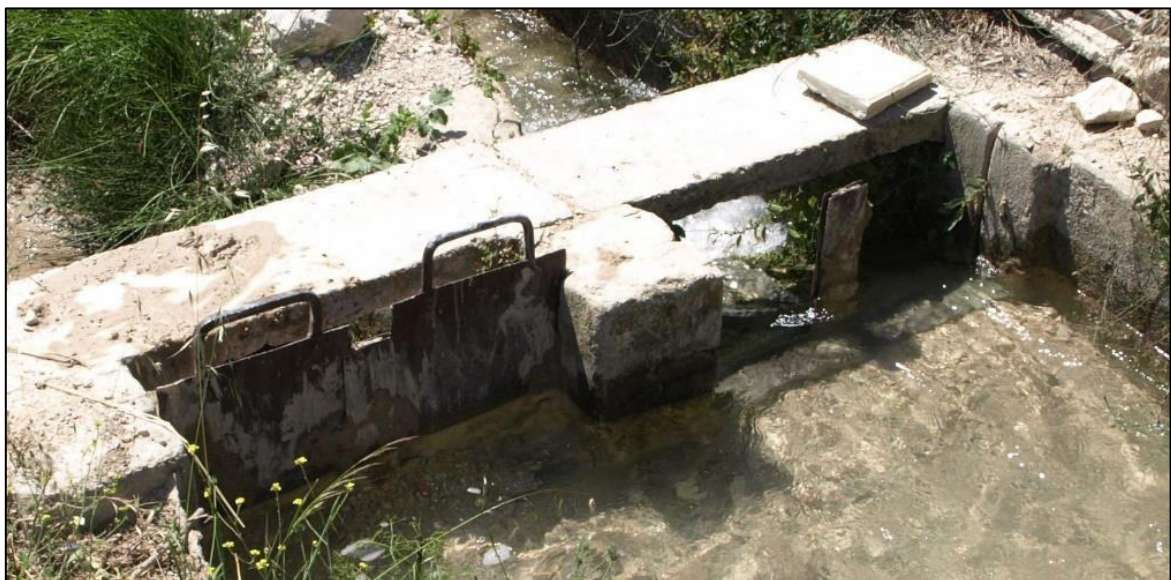
Fig. 4: The diversion of irrigation water is managed by a simple sluice system. This type of allocation technique is commonly used all over the Vega.
