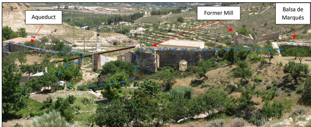
Fig. 9: Ruins of a former mill located below the Balsa de Marqués (for its location, see Fig. 10). The main technical elements of the water management are highlighted. The course of the irrigation water is highlighted by the blue dashed line.
