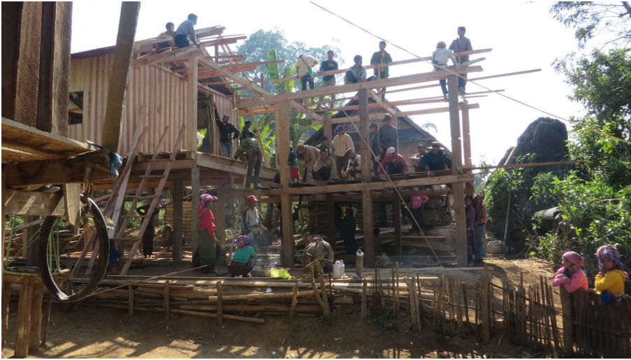
Figure 2 The erection of a wooden house in Pliya in 2015 Source: Photograph taken by the author [Colour figure can be viewed at wileyonlinelibrary.com ]
