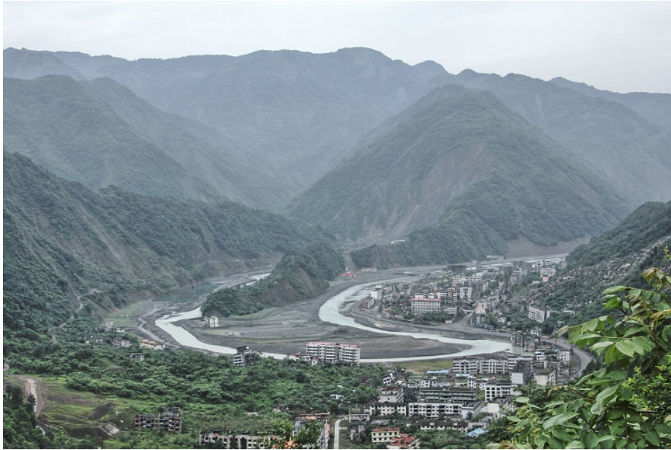
Figure 1.1: Landslides and rock slides triggered by the 2008 Wenchuan earthquake caused additional damage minutes after the earthquake. Photo by Martin Mergili
