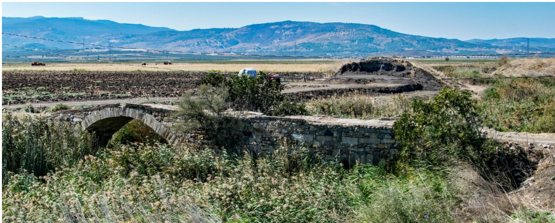
Figure 4. Hacismail Köprüsü (bridge 4) in the western lower Bakırçay Valley.
