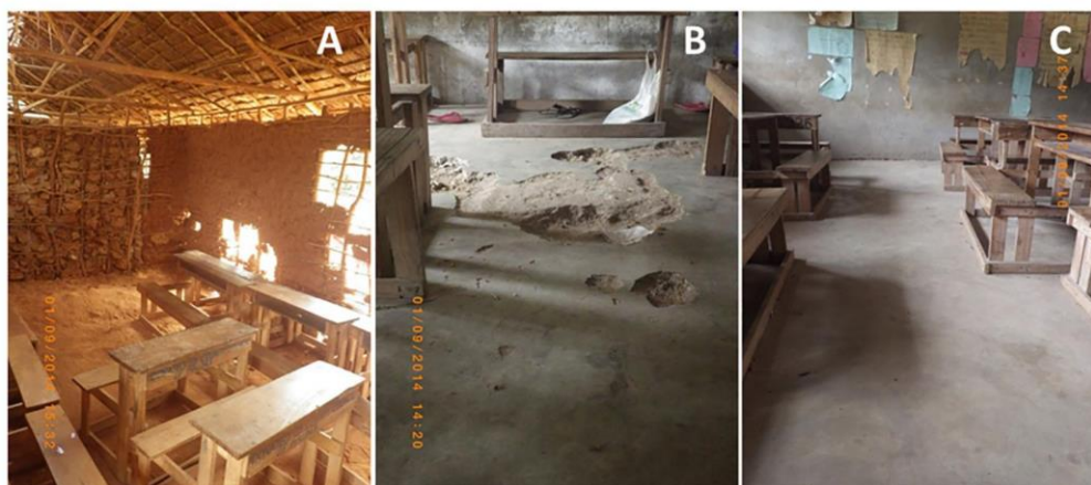
Fig 1. Examples of school classroom floors. (A) Natural sand/soil (MS2). (B) Cracked concrete (MS1). (C) Smooth concrete (MS1).
